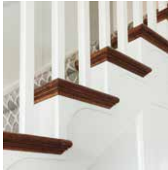
Open Tread Stairway
