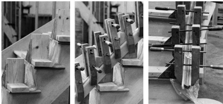
**Step 7** - Most handrails are ready to remove from the forms in 24-48 hours. However, when bending a very tight radius, it is advisable to allow more drying time. Take the rail assembly off of the bending forms and remove the bending mould. Remove the excess glue with a hand held belt sander.
